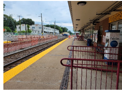
New tactile warning surface at Quantico
