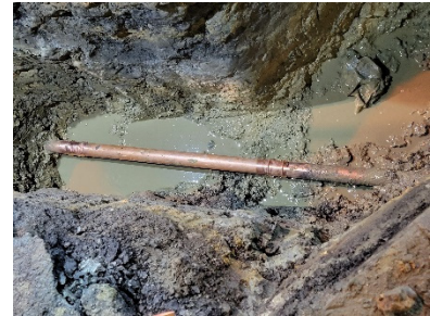
Water line repair at Quantico in progress
