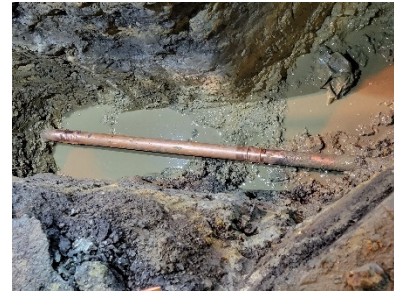
Water line repair at Quantico in progress
