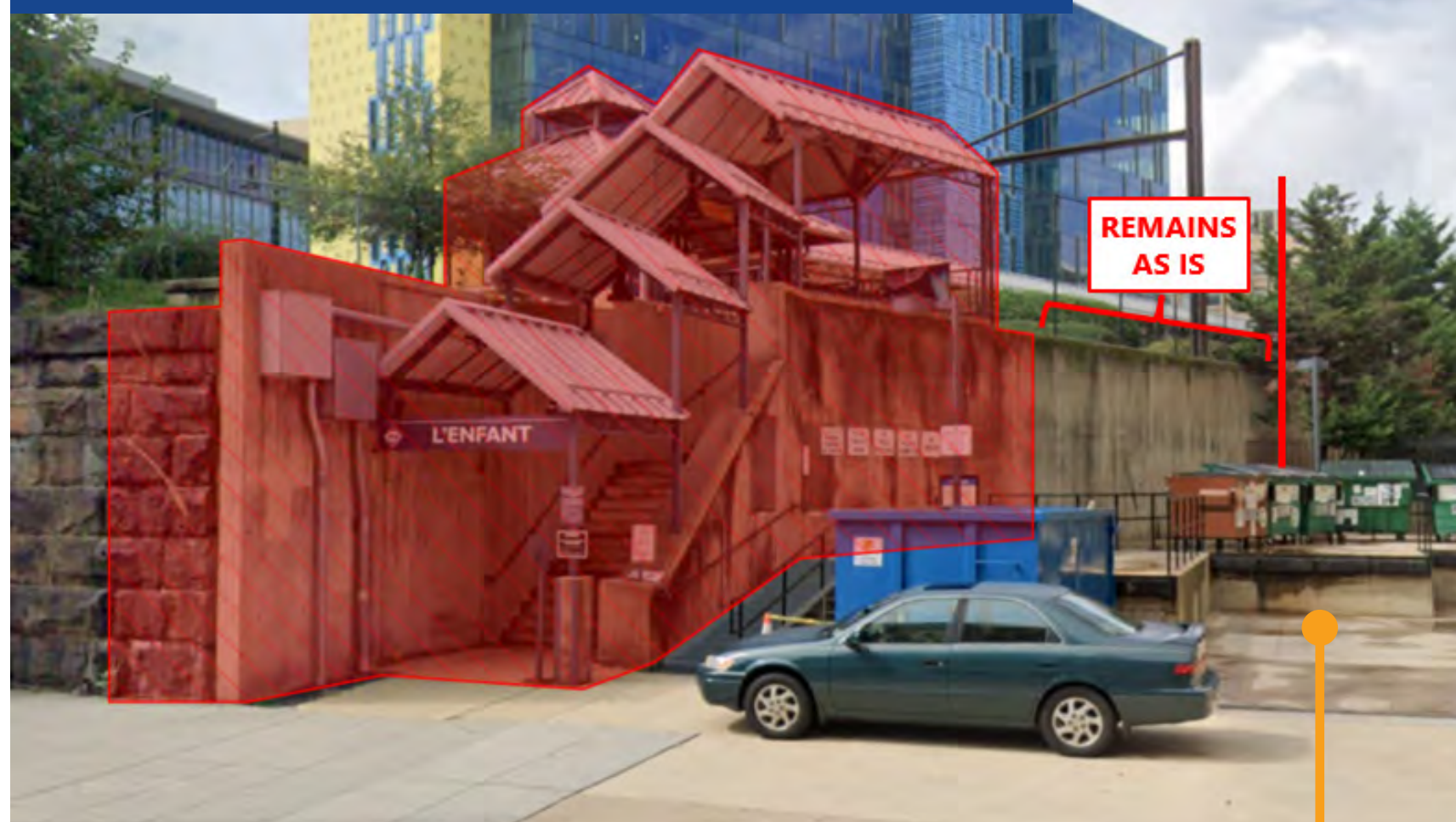
600 Maryland Ave loading area (Smithsonian office building)
