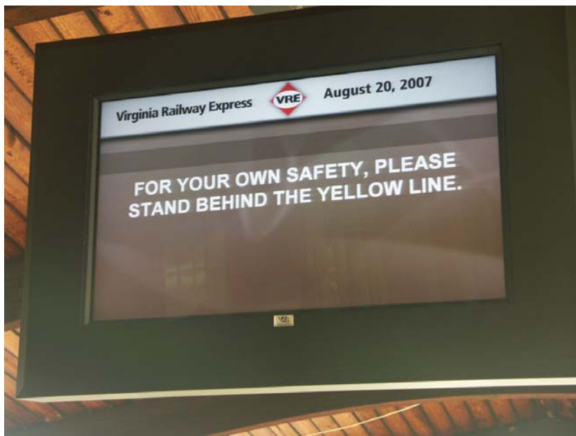
The new variable message sign at the Alexandria station: The darker rectangle underneath the VRE logo will show the train status information, while the bottom portion will be reserved for lengthier detailed messages, like the one shown here.
